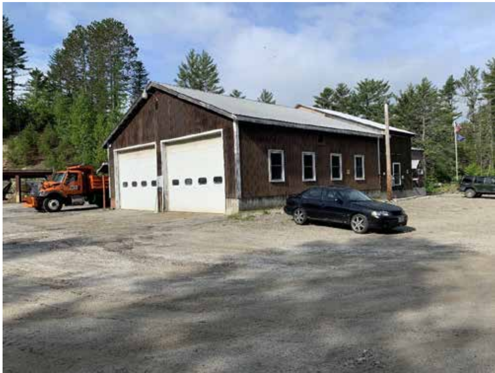
Truck bay exterior
