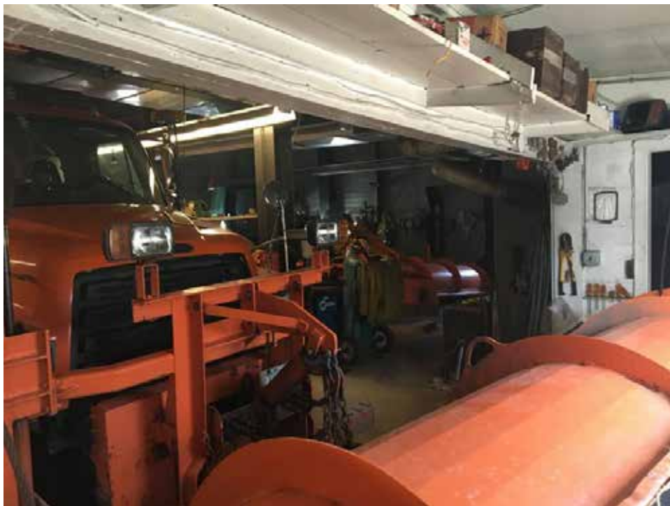
View of inadequate headspace over parked vehicle.
