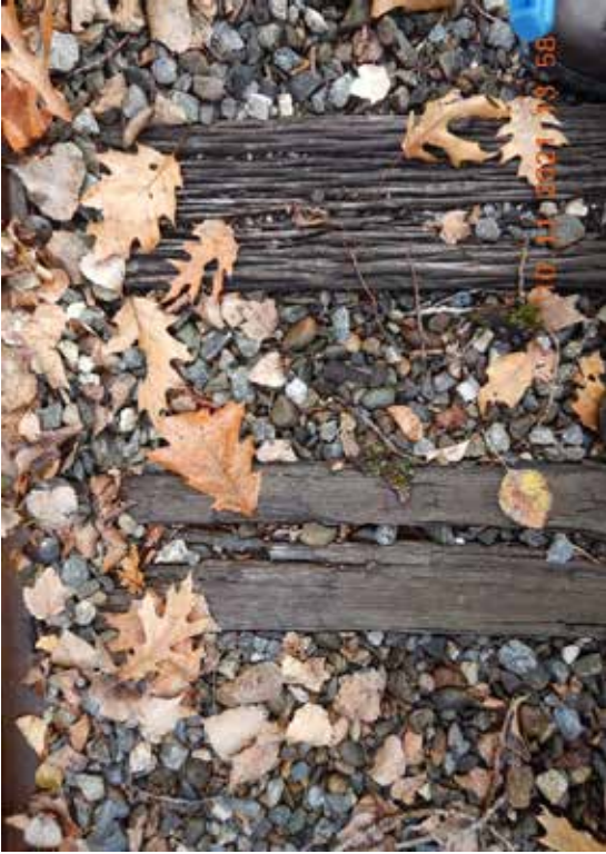
Concord-Lincoln Corridor, Concord Timber Railroad Tie Installed 1935
