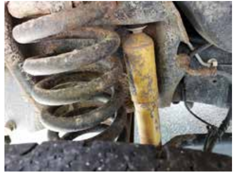
SCS: Undercarriage corrosion
