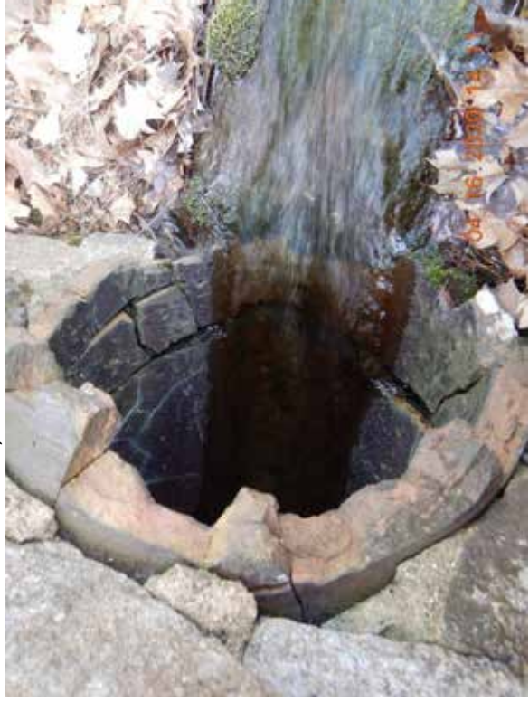
Concord-Lincoln Corridor, Laconia MP C34.91 Pipe Failure
