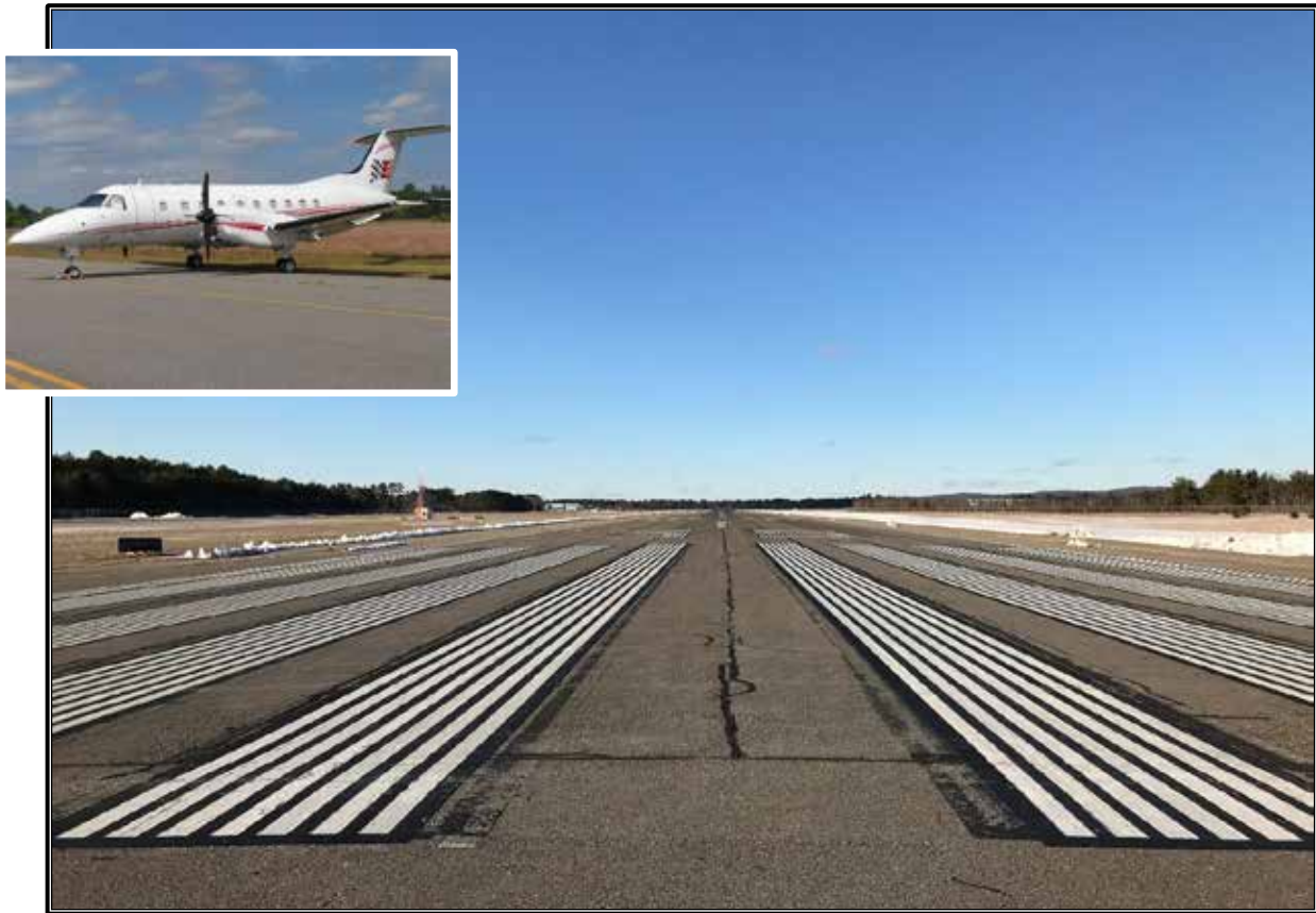
Figure 3: View of Concord Municipal Airport’s Runway 17-35.
