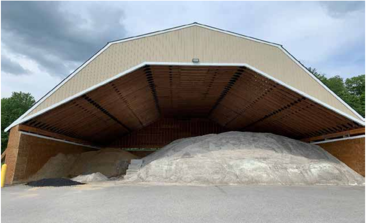
Combination of salt and sand in Franklin 211 section which is currently inefficient
